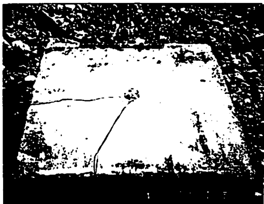
Fig. 4 Broken concrete block tested at 20°C
